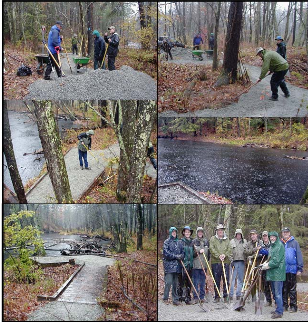
Chapter members fought the elements to spread stone dust on the pathways at the Universal Access Fishing Site in Townsend. The chapter constructed the two fishing platforms in 2000 and continues to maintain the site.
